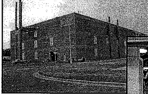
Solids Management Building
