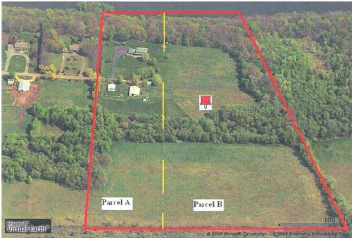
Attachment 6: Aerial photograph of Wicker parcels (outlined in red) and a portion of the two inholdings West (left) of the Wicker parcels that shows the buildings on those inholdings
