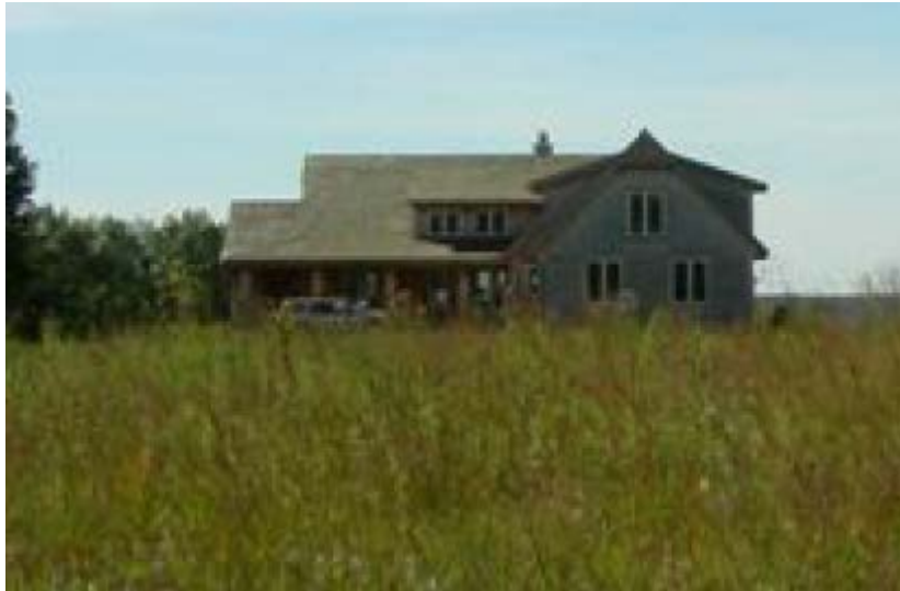
Figure 3: House and pole barns on Wells Fargo parcel
