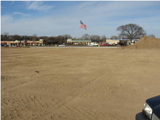
View from south-central portion of Property looking north at future building location
