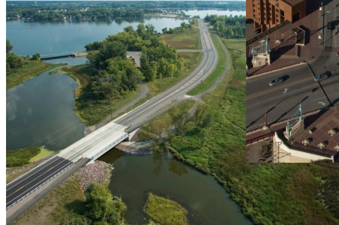
Anoka Co State Aid Hwy 54 (20 th Avenue in Centerville)
