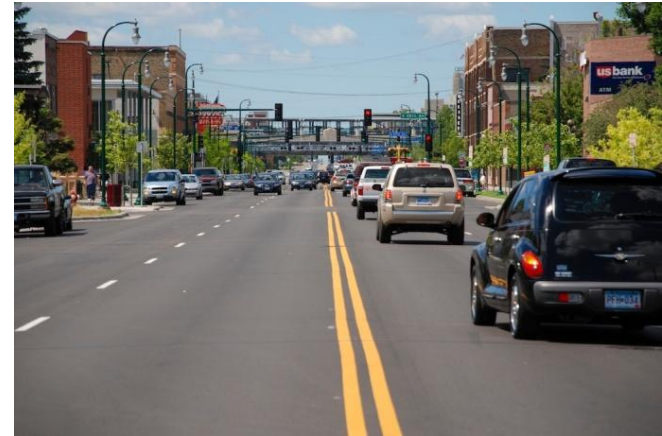
Hennepin Co State Aid Hwy 3 (Lake Street in Minneapolis)
