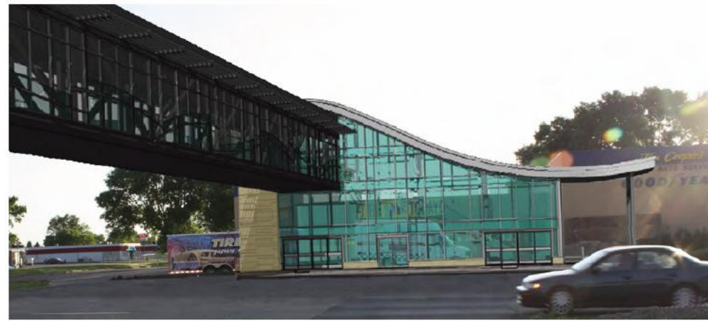
Southbound 147th Street Station Phase 2
