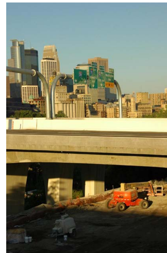
Figure 3-5: Bridge construction work is an investment priority mandated by the Legislature
