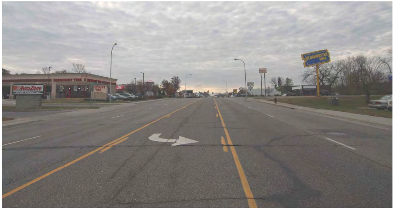
View of Southbound Robert Street Near Crawford Drive (Looking South)
