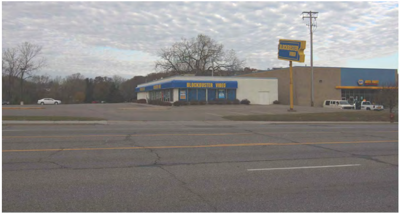
Proposed West Approach Area For Crossing At Crawford Drive (Looking West)
