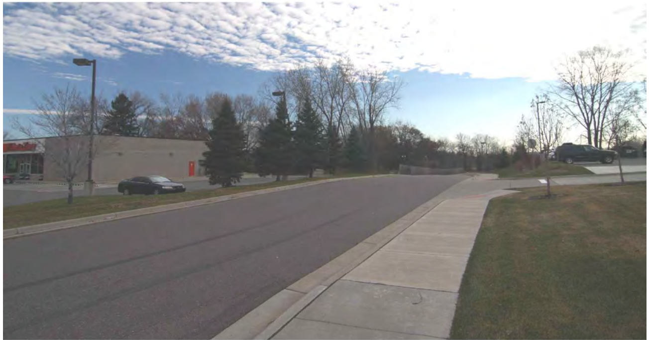
View of Eastbound Crawford Drive
