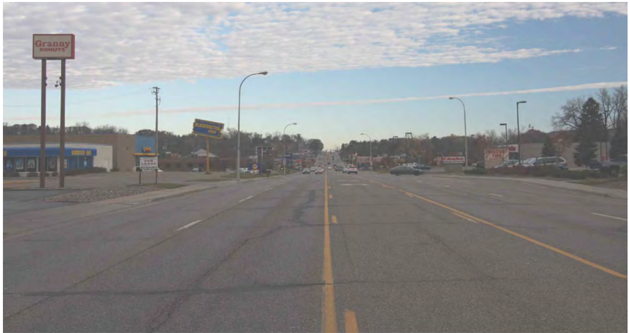
View of Northbound Robert Street Near Crawford Drive (Looking North)
